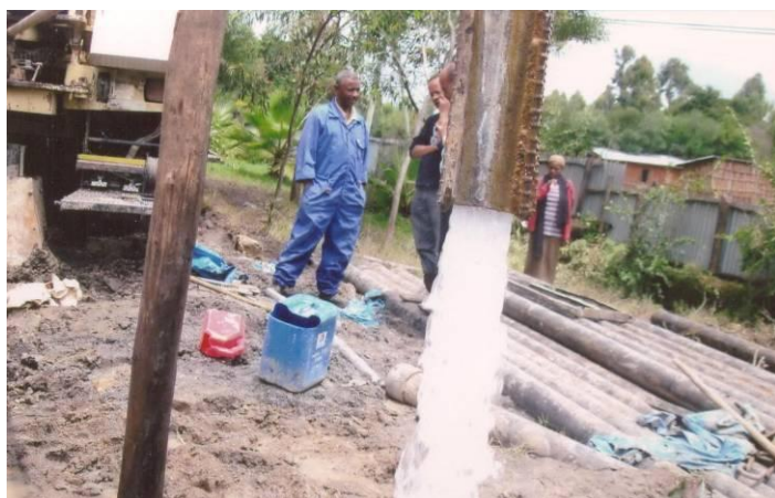
The new well in Ambo Town
