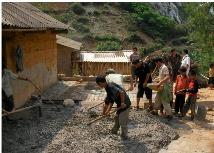
One of the new cisterns under construction
