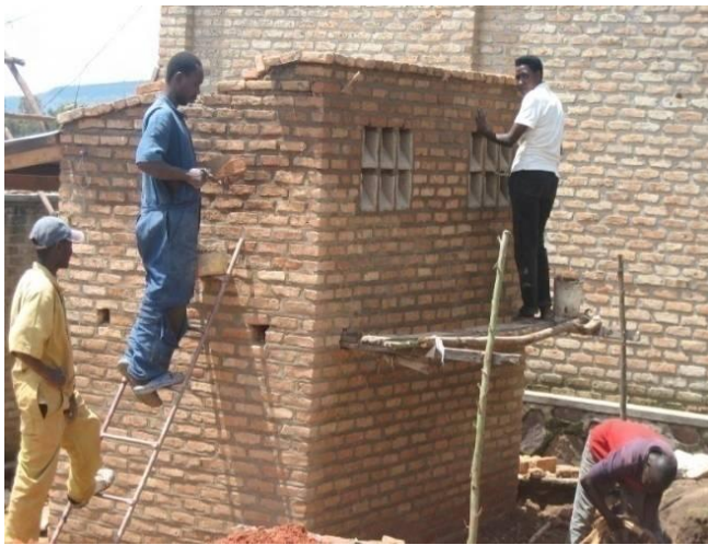
The new wash closet and shower under construction
