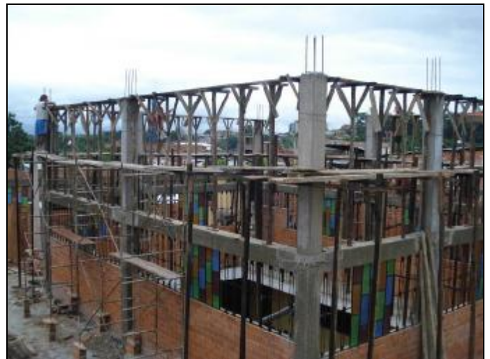
The Virgen María de los Remedios parish center under reconstruction
