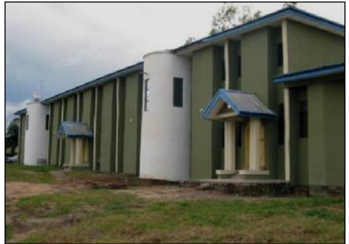
The newly completed postulancy building
