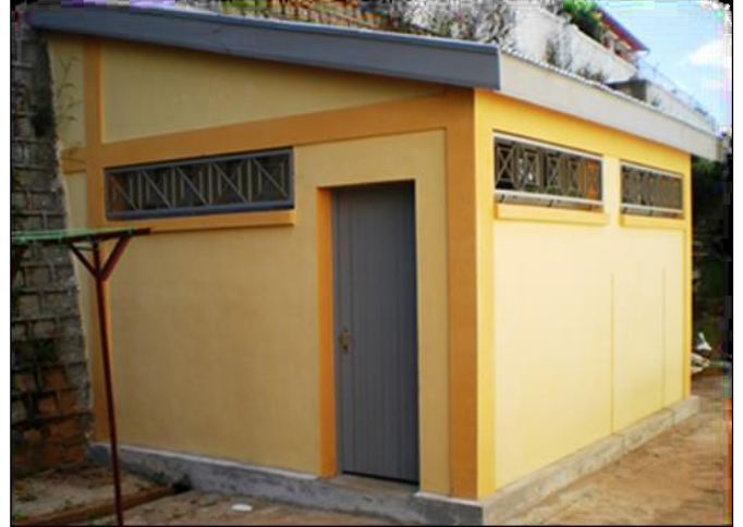
The new laundry at the Maison Saint Vincent
