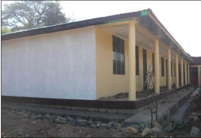
The new classrooms at SS. Peter and Paul School
