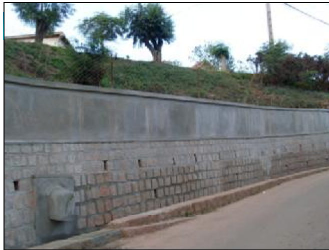
The new retention wall at the Maison Saint Vincent
