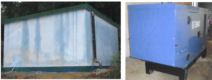
The new water storage facility and electrical generator at the Marillac Provincial House
