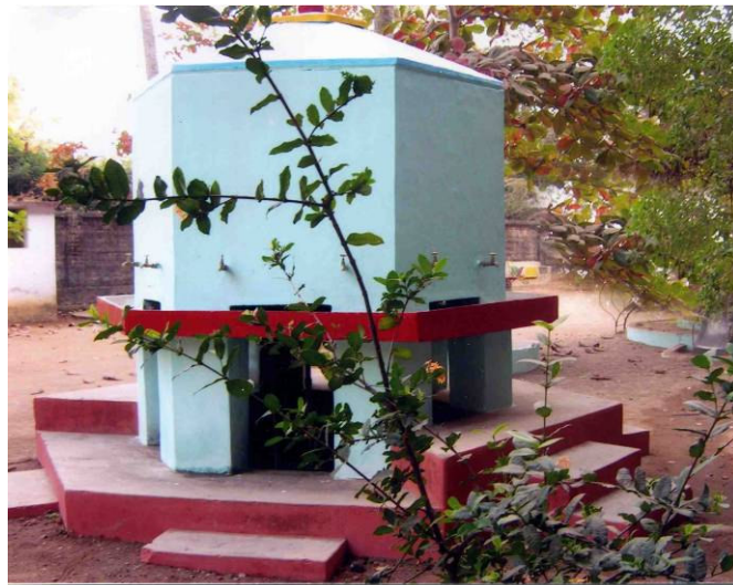
The new well at the Joshipur Hostel in Orissa
