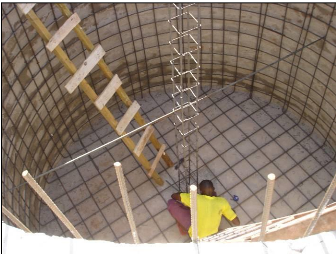
The new water storage tank nearing completion
