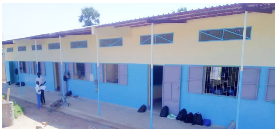
New classroom block
