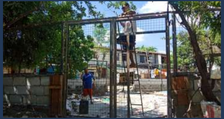
Philippines: Vincentian Family Children's Playground construction project.
