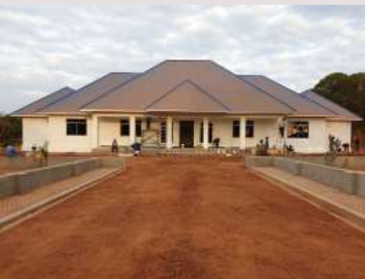
Tanzania: Expansion of the Regional Administration House and addition of 20 guest rooms for retreats and seminars.
