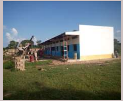
Chad: Construction of a 'three- classroom' block for Lycée Collège St. Jean-Baptiste de Bebalem.
