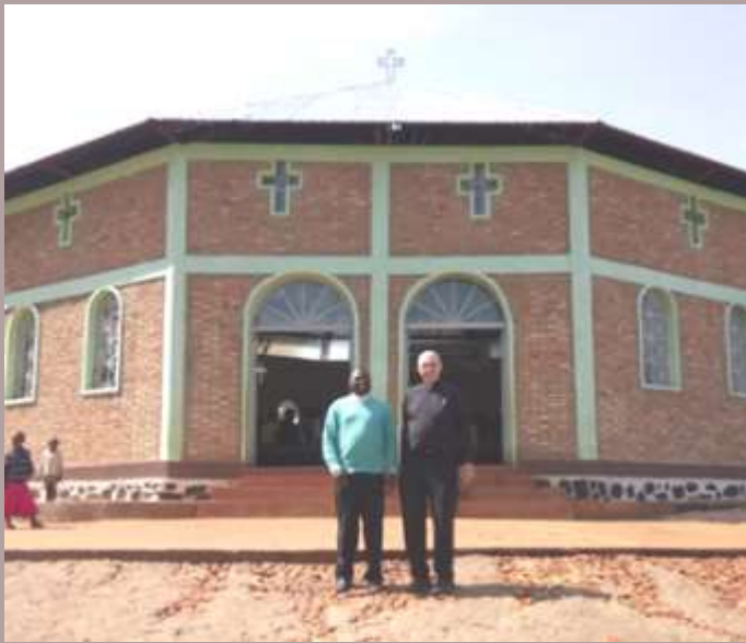
Burundi: New Church Construction at Rabiho.
