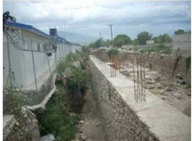
The retaining wall under construction by the school
