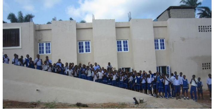
The new inclusive school hostel and its students
