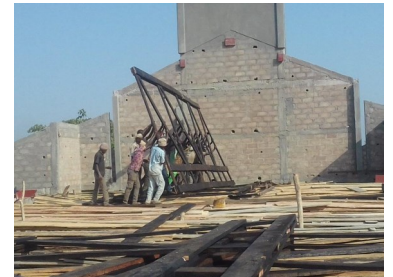
Raising the Supports for the Roof
