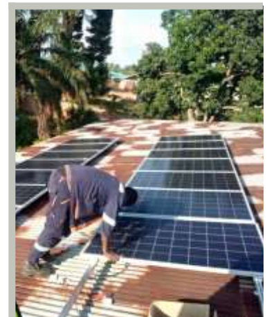
Rooftop install of solar panels for the Parish offices
