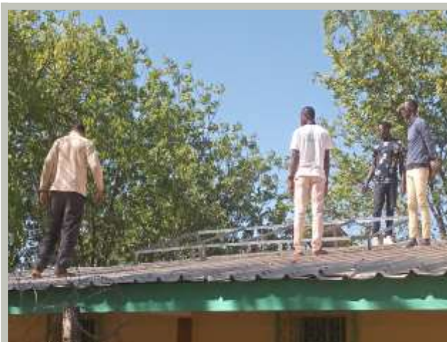
Installing the rooftop solar panels
