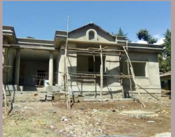
Ethiopia: Construction of new presbytery for the catholic community of Kochi of the Apostolic Vicariate of Nekempte
