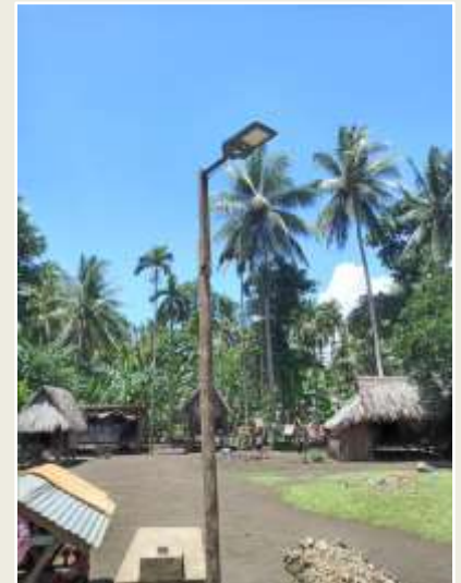
New solar streetlights in Papua New Guinea
