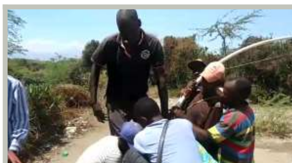
Work on the well begins
