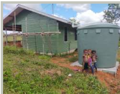
Pictured right: finished building and water tank.
