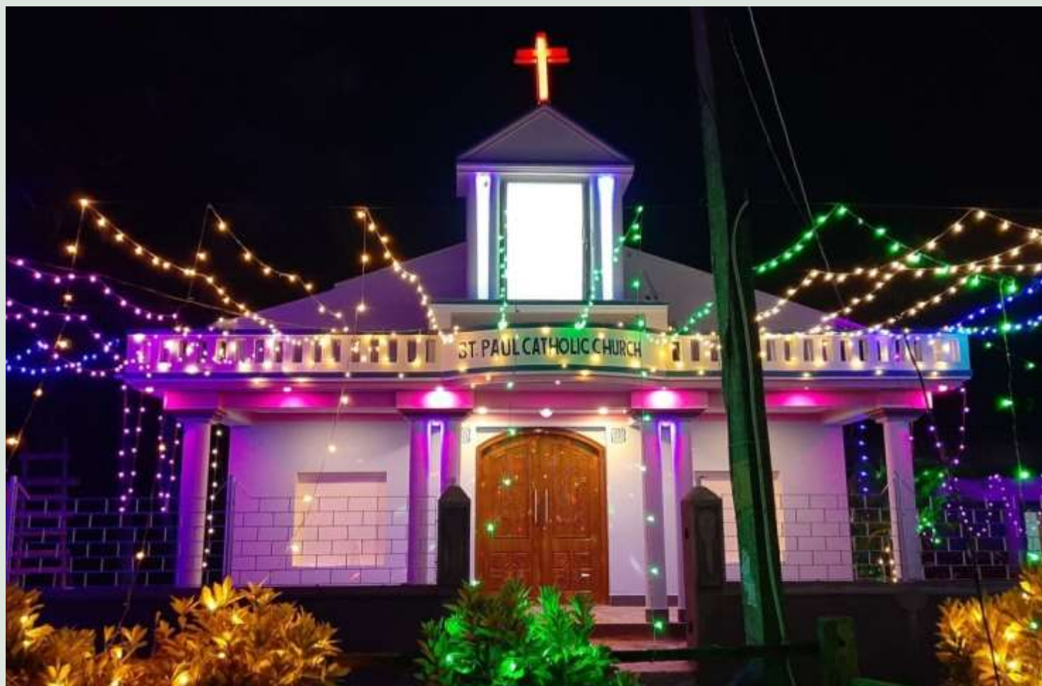
Pictured: Extension and Renovation of St. Paul's Catholic Church at Canning in the Diocese of Baruipur, W. Bengal, India
