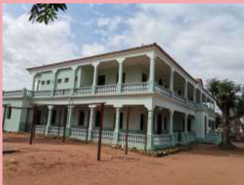
Renovation of the Institute of Agriculture High School in Magude, Mozambique
