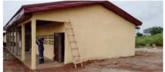
Above: Construction nears completion
