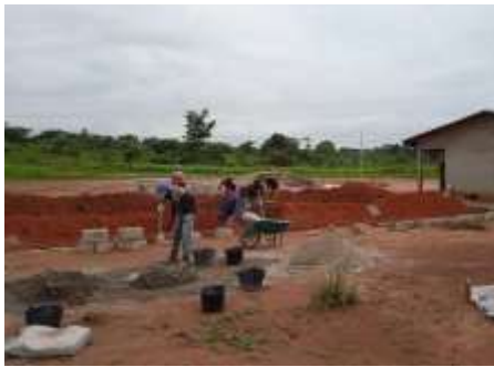
The beginning of construction of new classrooms
