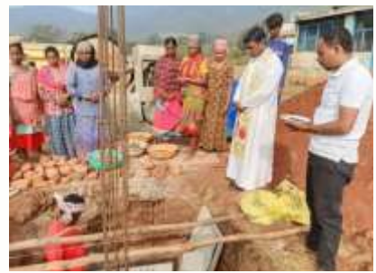
Renovation of Dukuma Church, India
